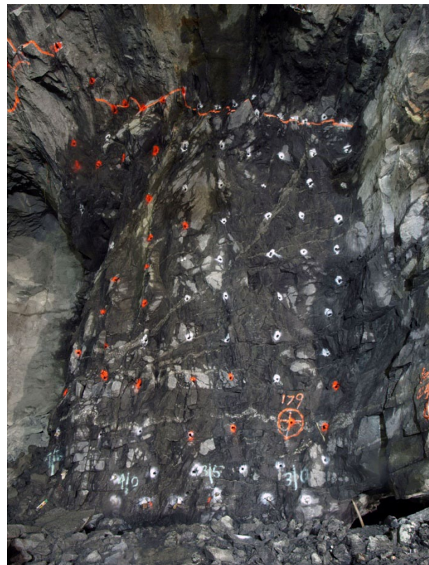
Figure 13 - Isoclinal recumbent folds of early SE-dipping foliation in Hartland formation (OCh) outlined by granitoid sills (g) with gently inclined penetrative foliation. Recrystallization during folding and shearing produces penetrative mica foliation (Feature 10.) that has formed parallel to compositional layering. Gently inclined foliation joints are prominent discontinuities ( J_1 ) and have formed parallel to the foliation and parallel compositional layering. These are intersected by steep NE-trending ( J_2 ) and NW-trending ( J_3 ) joints and faults producing overbreak seen at top of image. (Digital image taken 19 December 2012.)
