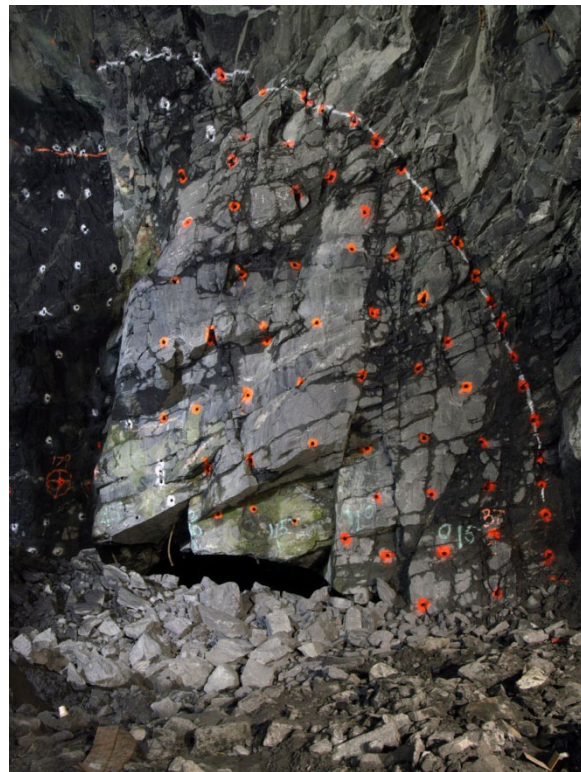
Figure 14 - Geological map and southward view digital image of west slash of North Cavern below 85th street in NYC. Note the internal structure dominated by internally sheared gentle SE-plunging isoclinal recumbent folds of early SE-dipping gently inclined foliation in Harland formation (OCh). Recrystallization during folding and shearing produced penetrative mica foliation (Feature 13.) that formed parallel to transposed compositional layering. Gently inclined foliation joints are prominent discontinuities ( J_1 ) and have formed parallel to the foliation and parallel compositional layering. These are intersected by steep NNE-trending ( J_2 ) and NW-trending ( J_3 ) joints and faults producing overbreak (light green shading). (Digital image taken 19 December 2012.)
